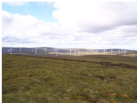
Overview Paul's Hill Windfarm with 28 turbines in operation
