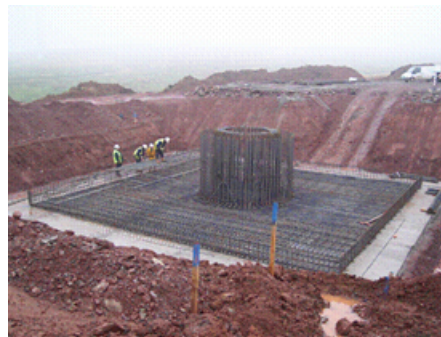
CRYSTAL RIG extension (additional five turbines)
